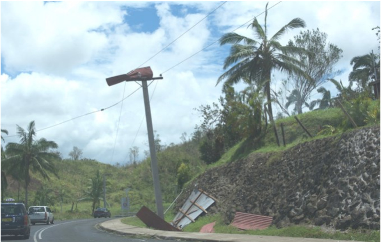
The Emergency Telecommunications Cluster deployed specialised staff to assess damage to communications systems. Photo: WFP / Francesca Ciardi
