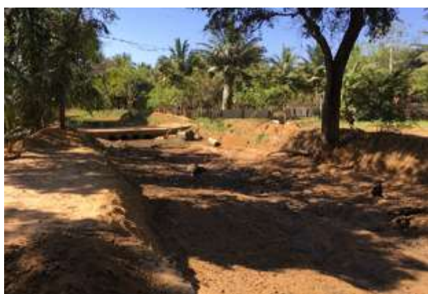
Image 3.6. A cleared drainage channel that feeds into a minor tank (a few kilometres away) in Mudkompan
