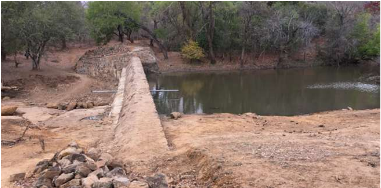
Image 3.3. Matande weir downstream from a dam
