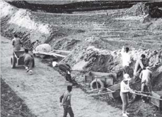
WFP beneficiaries constructing a water storage dam in the Anseong watershed
