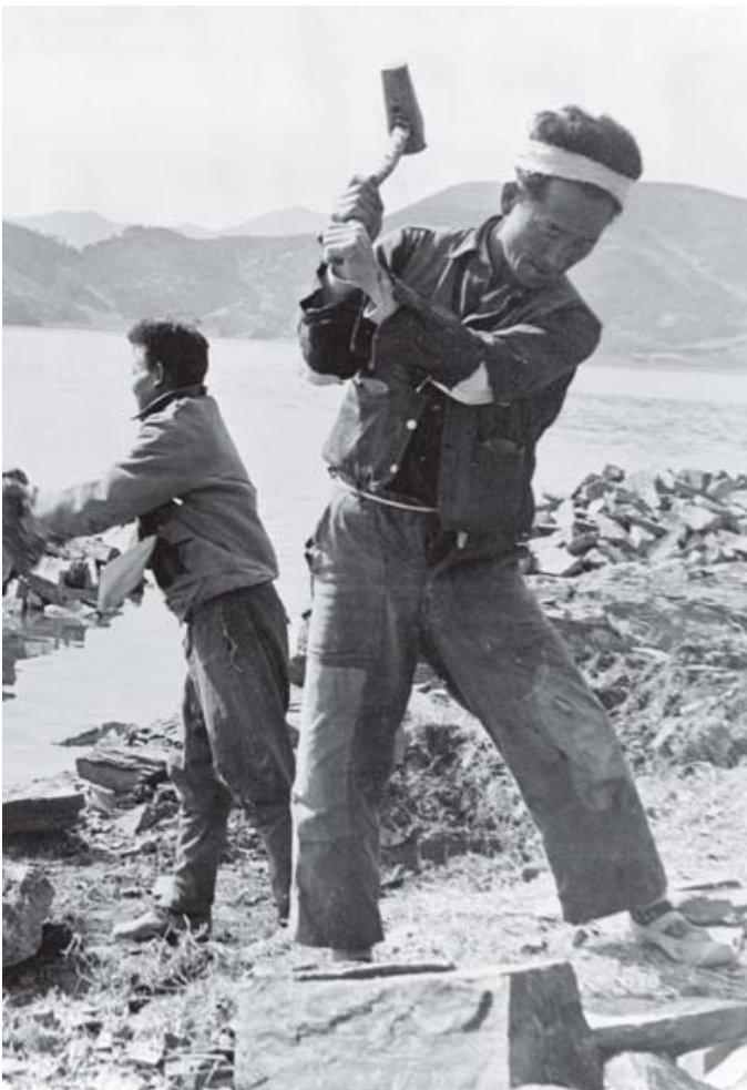
Laborers working at a land reclamation site
