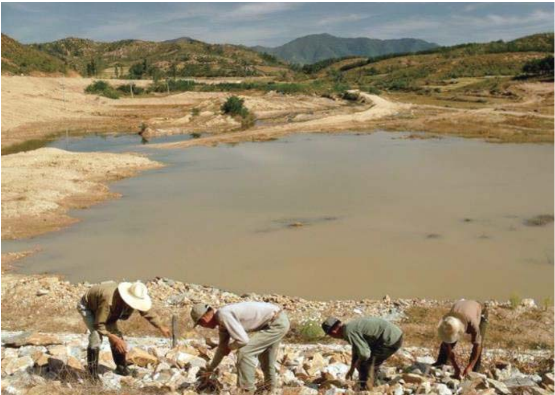
Workers at a construction site for a water storage dam
