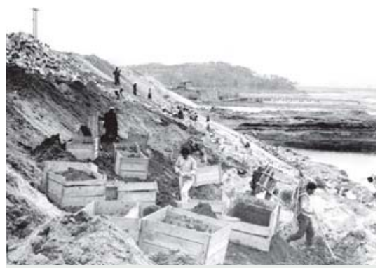
Construction site of an embankment at Wangsukcheon in Namyangju
