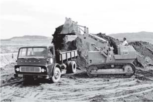
Removing sand to construct a fishery in the Nakdong river basin
