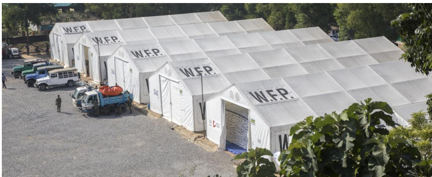
Ukhiya logistics hub , serving government and humanitarian partners in Cox's Bazar. A large humanitarian staging area, to respond to major natural disasters, is planned.
