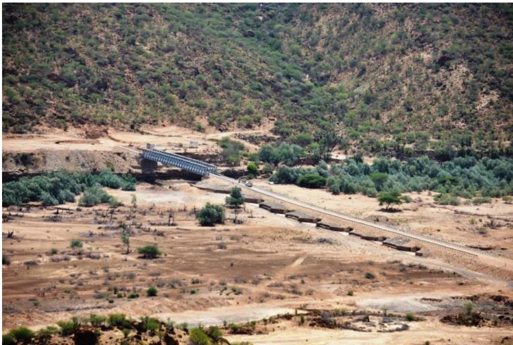
Figure 66 Completed Geeldoh bridge
