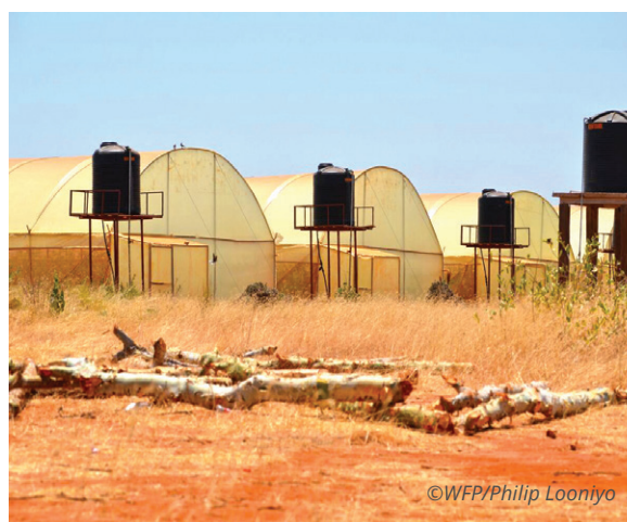
Small-scale irrigation projects in Qara, Wajir West. WFP provided hybrid irrigation infrastructure consisting of solar systems and pump sets to convey water to farms.
