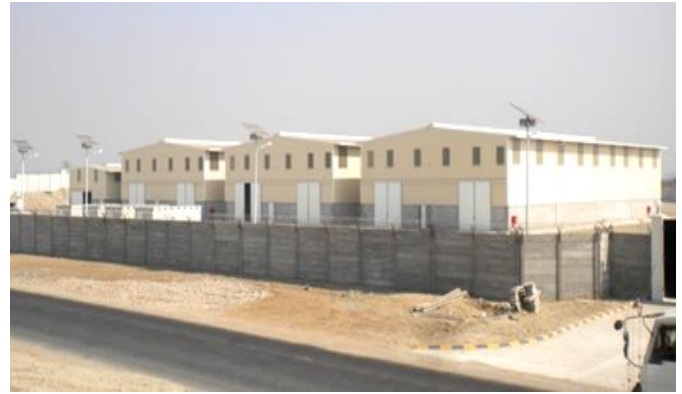
Humanitarian Response Facilities (HRF) in Muzaffargarh.
