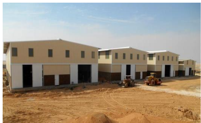
Humanitarian Response Facilities (HRF) in Hyderabad
