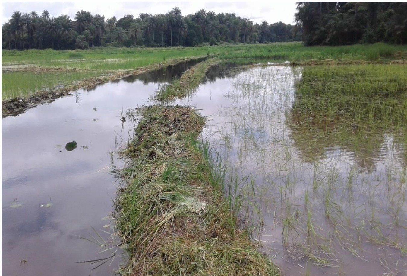
Figure 1: Lowland irrigation structure damaged by heavy rainfall, Roline, Maforki chiefdom, Port Loko district (Sulaiman Coker, WFP)
