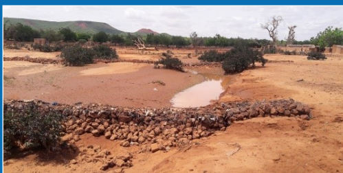
Check-dams for gully control, soil and moisture retention.
