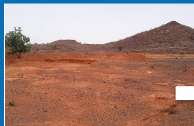
Construction of the pond during the dry season.
