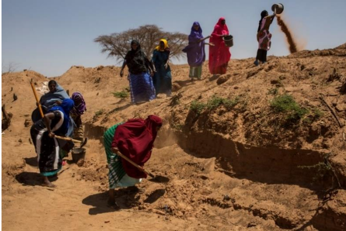
Picture 8: Picture 6: Communities working in desilting and expansion of water catchments in Beerato village Odweyne – ©FAO/WFP/Will Baxter
