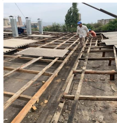
Renovation process of a school bakery roof in Spitamen District of Sughd Region with the support of WFP within its School Feeding Programme. ©WFP
