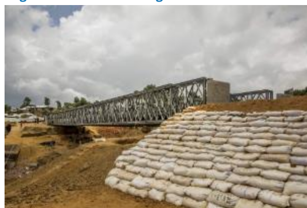
Figure 8: Mabey Modular Bridge: a rapid-build, pre-engineered modular bridge
