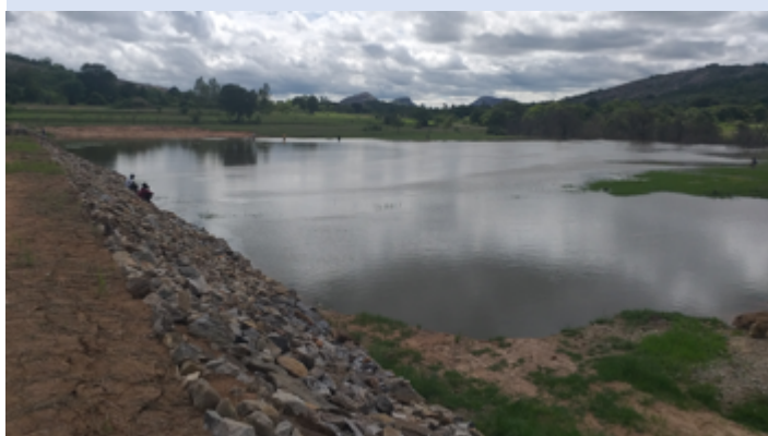
After the intervention
