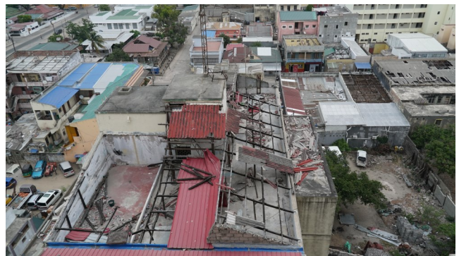
Hospital destroyed by TC Idai in Beira city, capital of Sofala province
