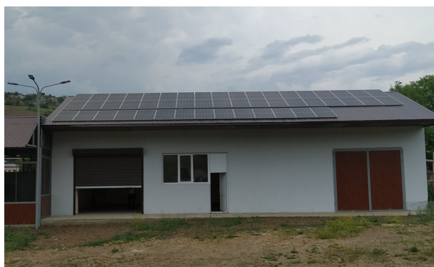
Collection centre powered by solar energy
