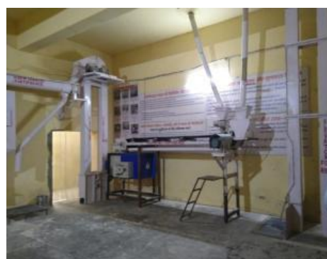
Fortification equipments at mill
