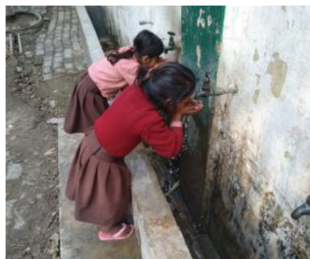
Drinking water facility at school
