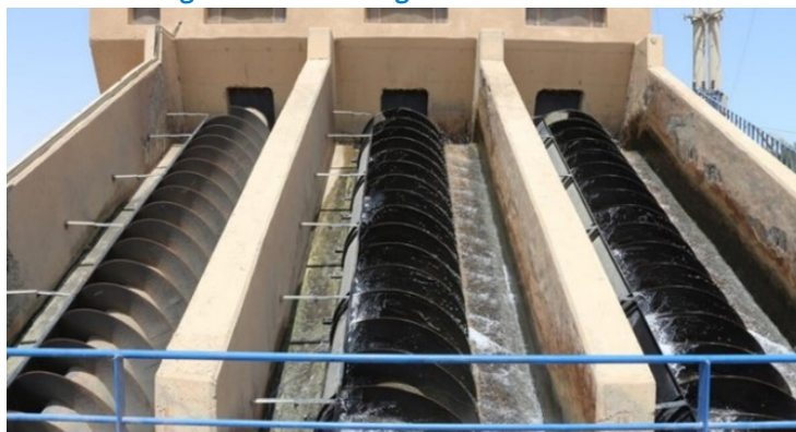
Figure 17: The lifting station in Sector 5
