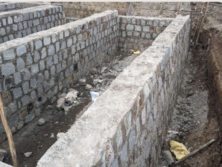
Construction works of the Eka Kotebe hospital. Photo: WFP/Ethiopia Country Office
