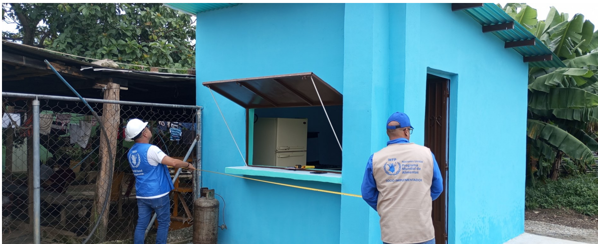
Rehabilitation process of school kitchens in Venezuela. Photo: WFP/Venezuela Country Office
