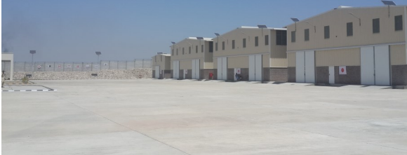
Construction of the humanitarian response facilities in Pakistan.
