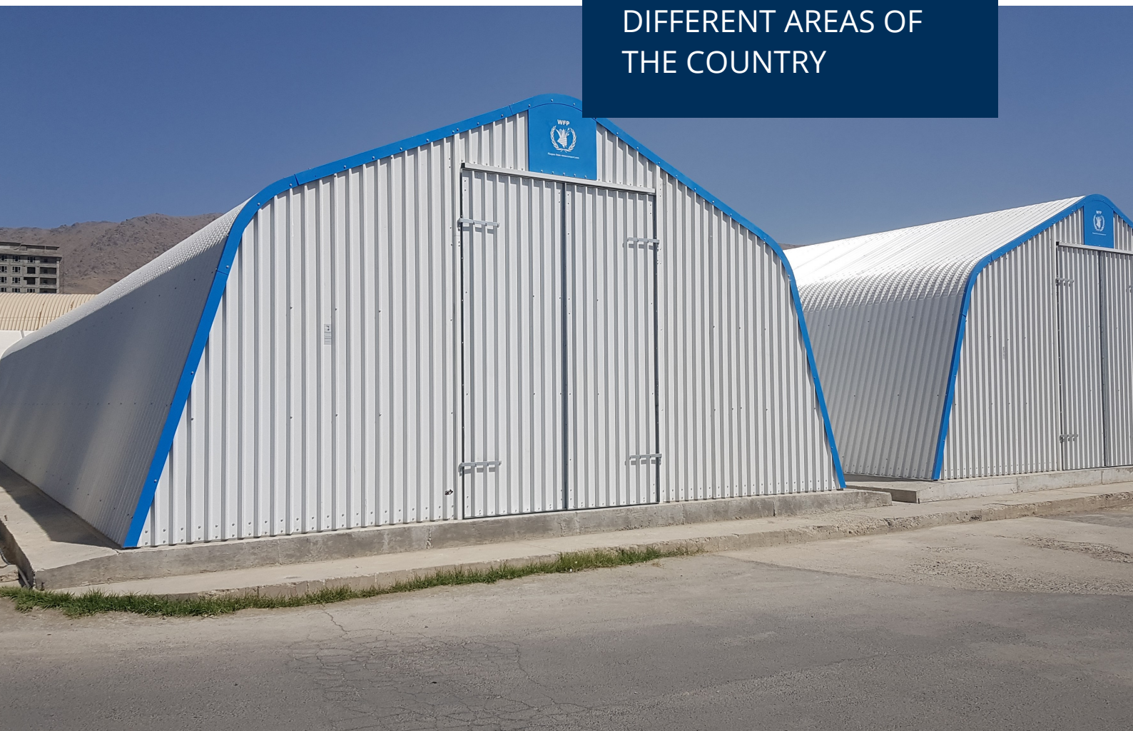
Warehouse upgrades in Kabul. Photo: WFP/Afghanistan Engineering team
