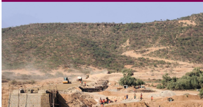
Geeldoh Bridge in Ethiopia under construction. Photo: WFP/Country Office Engineering team
