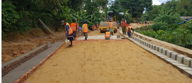
Road rehabilitation works in Cox's Bazar. Photo WFP/Country Office Engineering team
