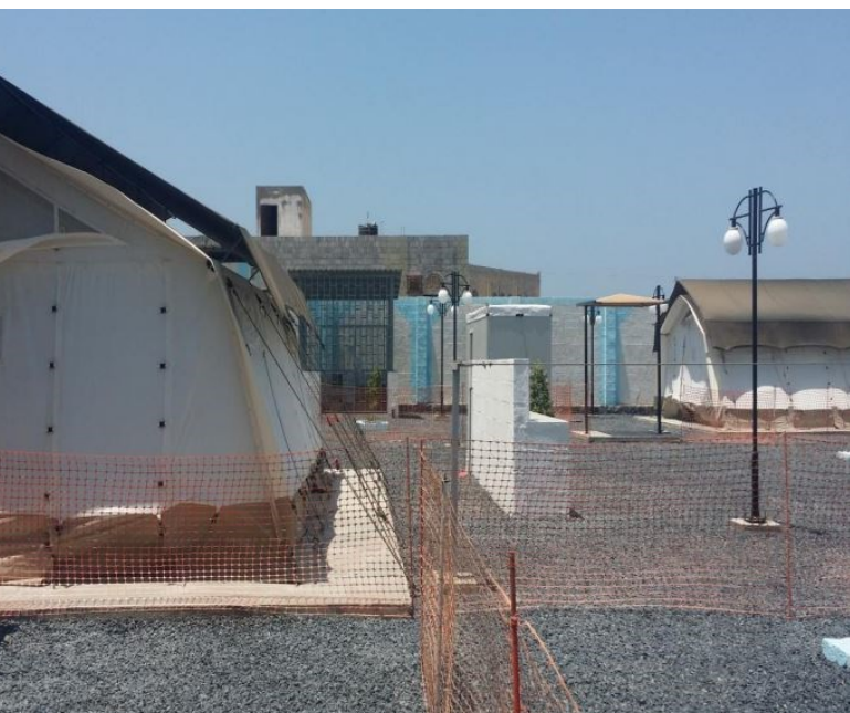
Al Salif Medical Centre in Yemen. Photo: WFP/Country Office Engineering team
