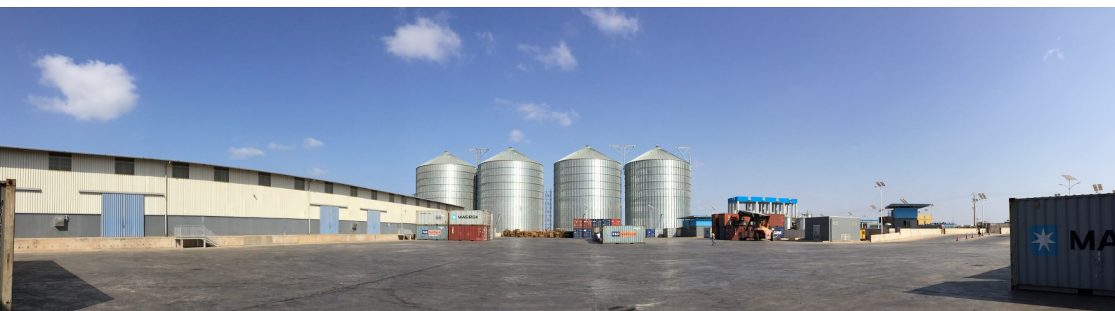
Humanitarian logistics hub in Djibouti. Photo: WFP/WFP Engineering
