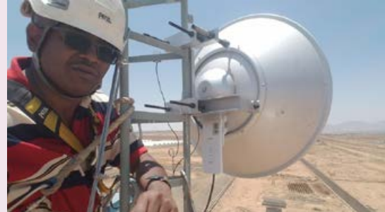
"We set up this 18m radio mast by hand, because no crane was available and we had time to concentrate."
