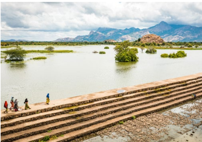
Rehabilitated dam (Guera, Chad)
