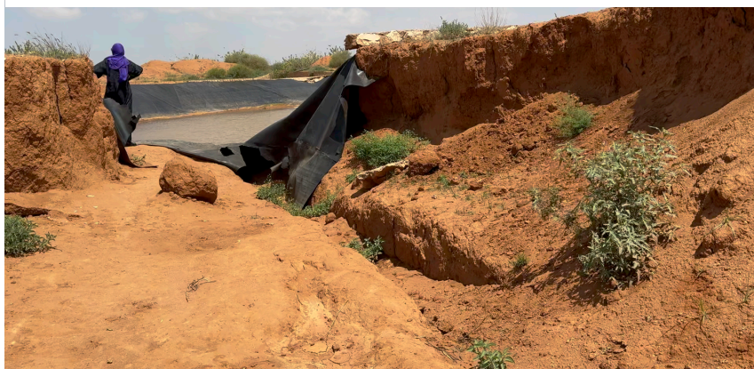
Figure 6: "Some of the water catchment plastic was in disrepair." Water catchment area, Galooley
