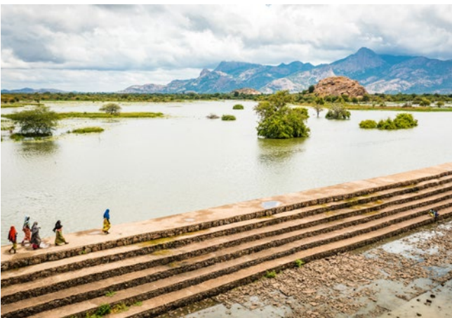
Rehabilitated dam (Guera, Chad)
