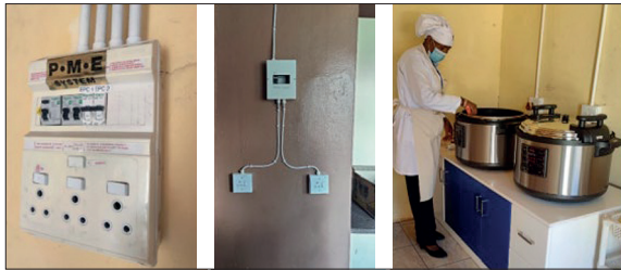
Figure 1: Adding new circuit breakers and electric sockets in the school kitchens
