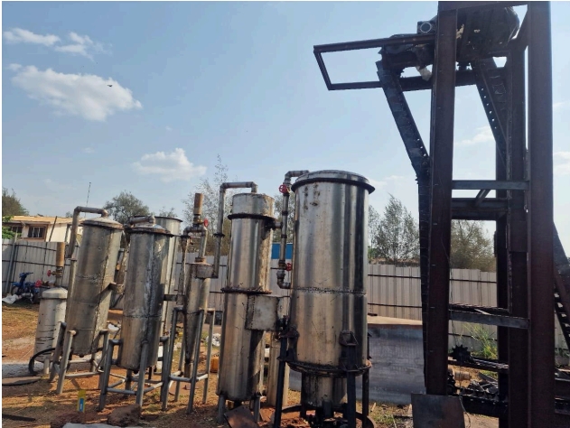
Coupling and quality testing of rice paddy parboiling and dryer system in Nigeria. | Photo: BEBEQUE
