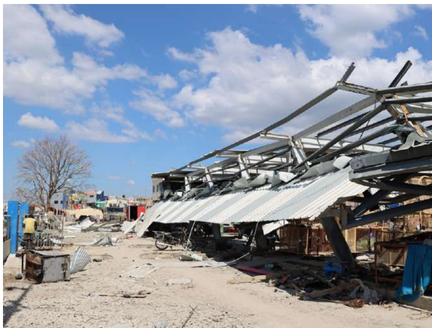
Clearing of debris in the centre of Black River, one week after catastrophic Category 5 Hurricane Melissa made landfall, Jamaica.
