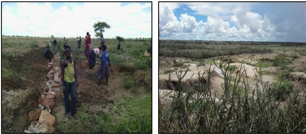
Photo 5: Construction of check dams using rocks and reinforcement with milk bush in Kotido
